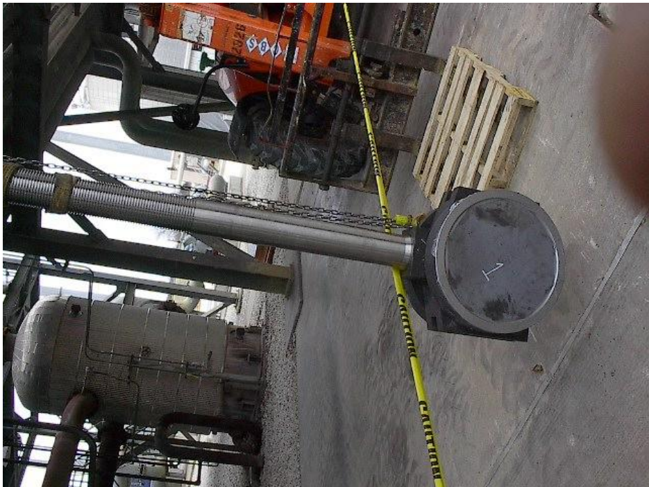
Stem and discs ready for assembly
